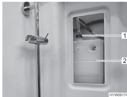
Fig. 211 Compensator reservoir (hot-water heater)
